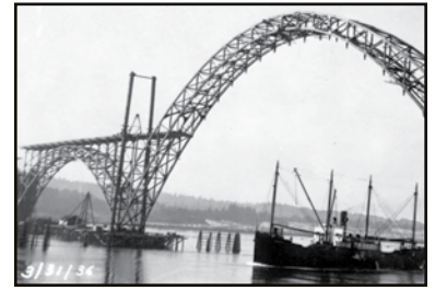
Yaquina Bay Bridge five months before opening to traffic.
